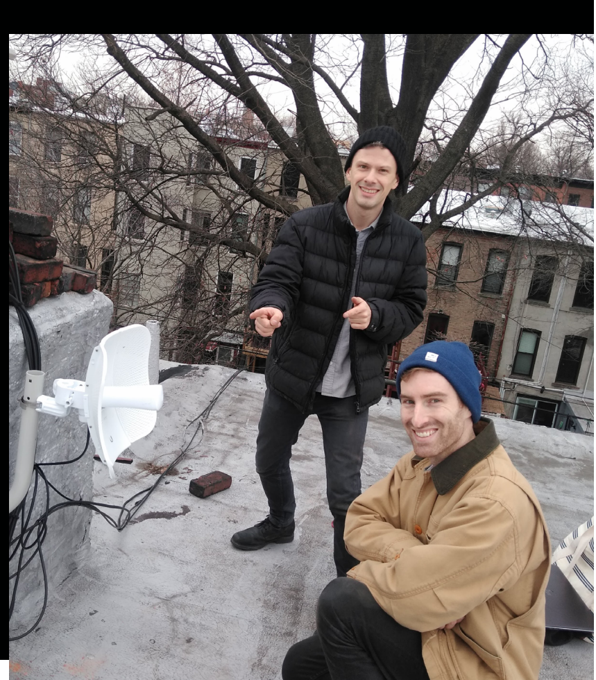
Volunteers successfully installing a Litebeam in Brooklyn.
